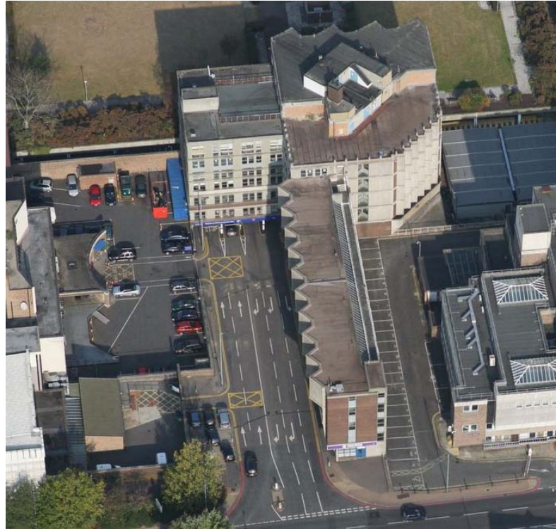
Aerial view of southern elevation (including access under the existing building to the public car park from the Barclay Road Ramp)
