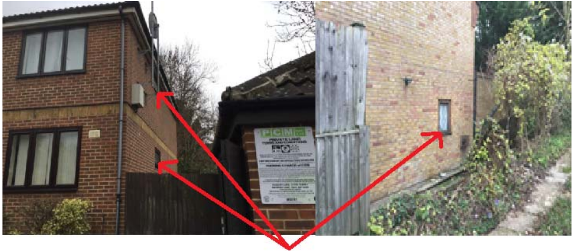
Image I – Image and Location of Windows that Fail BRE Guidelines
